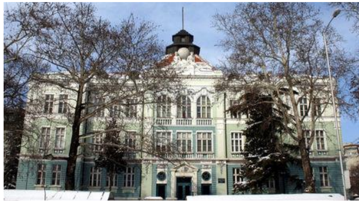
Fig. 5. Digital image of the facade of University of Economics – Varna
