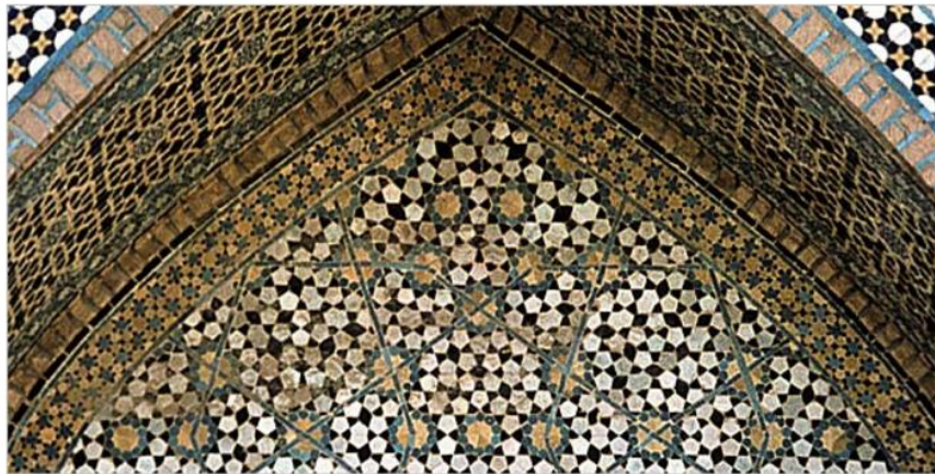
Figure 57: Mosaic Sophistication - A quasi-crystalline Penrose pattern at the Darb-i Imam shrine in Isfahan, Iran. Credit: Dudley and M. Elliff.
